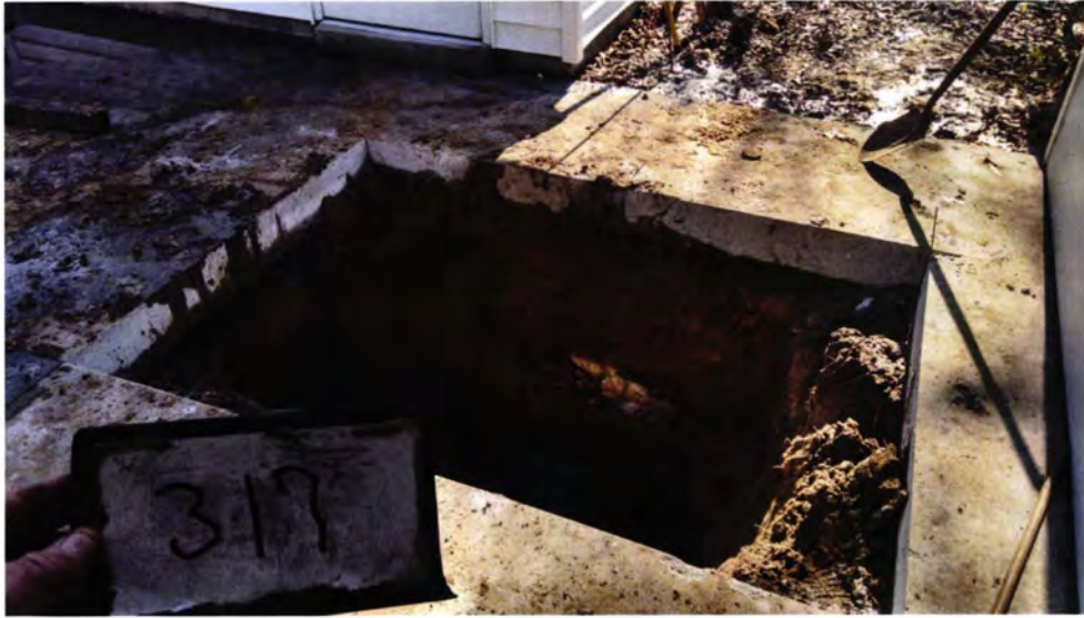
Picture 3: UST 317Ash's excavation.
