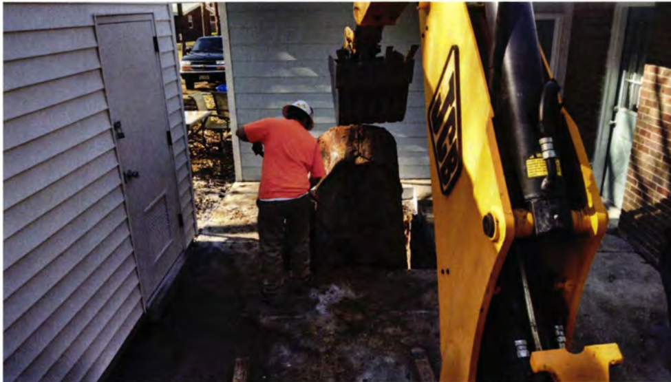
Picture 2: The tank being lifted from the excavation.
