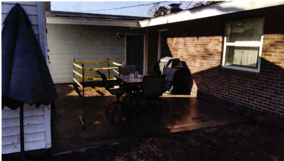
Picture 4: Site at completion of tank removal.
